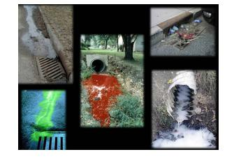
An illicit dischage is any discharge to the storm sewer system that is not composed entirely of rain water or ground water.
